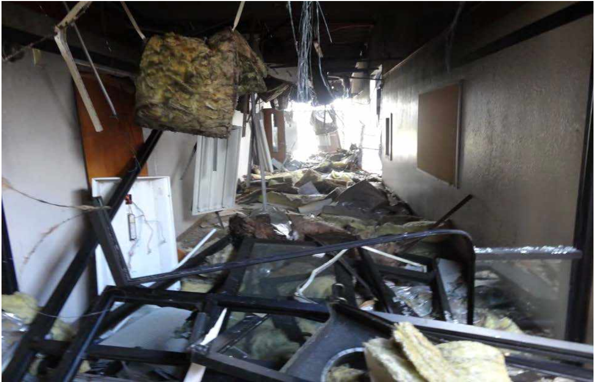
[그림 18] WS North Hallway, Looking Toward Northeast Exit Door (Source: ABS Consulting)
